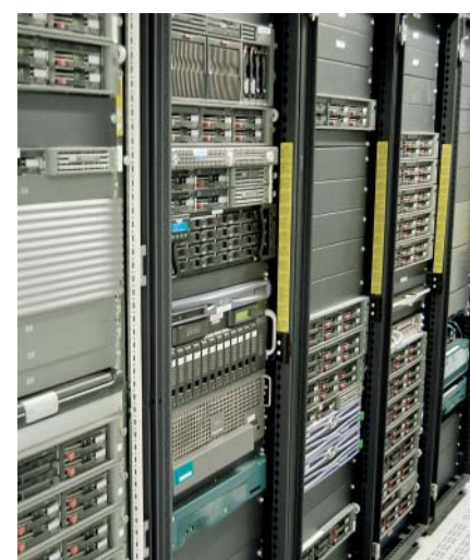
The Aareon IT Service Centre was upgraded in 2005.
